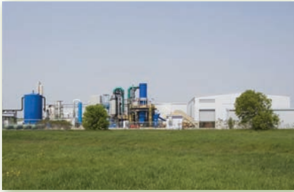
Converting waste to clean gas and valuable products without emissions
